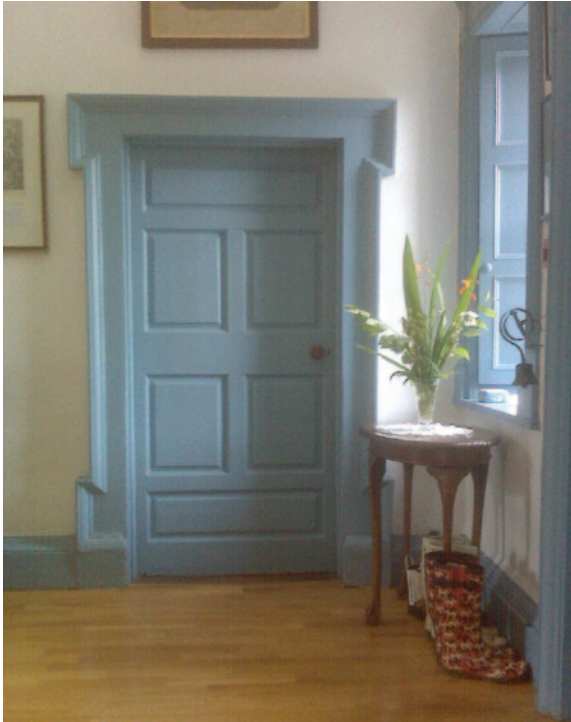
Detail of entrance hall, door with shouldered architrave
