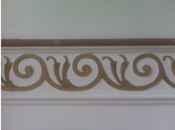
Staircase, frieze with Vitruvian scroll at first-floor level
