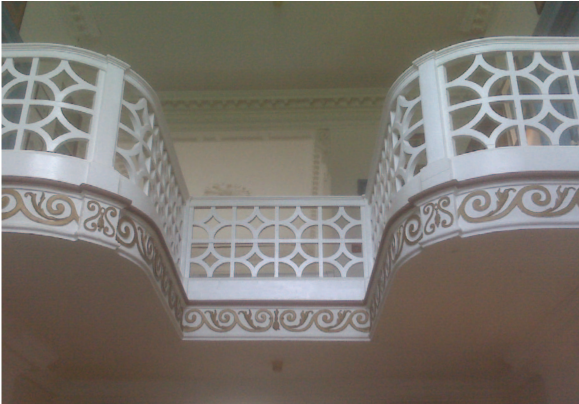
Entrance hall, curved balconies at first-floor level
